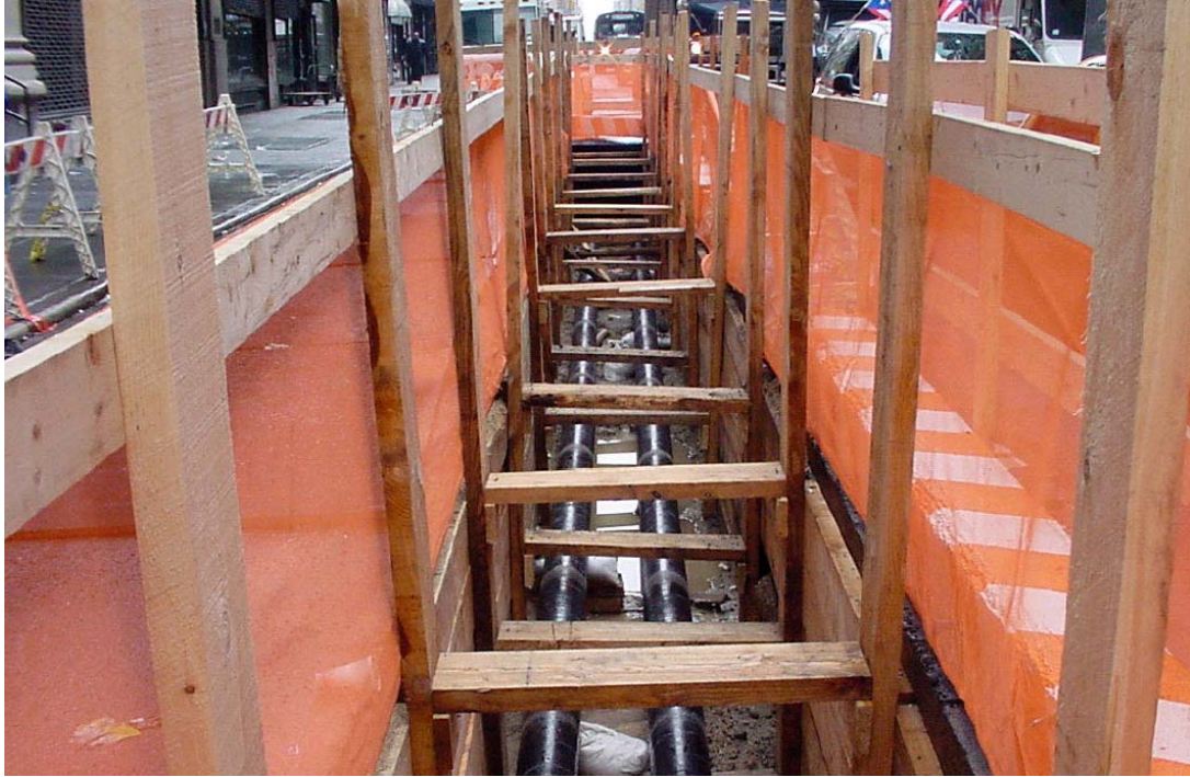
Figure XII.1.3.1 Trench Having Two Conventional Cables West 30 th Street near Fifth Ave. in New York City
