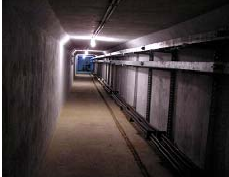
Figure XII.1.3.2 Cable Tunnel in which Cables Have Not Yet Been Installed
