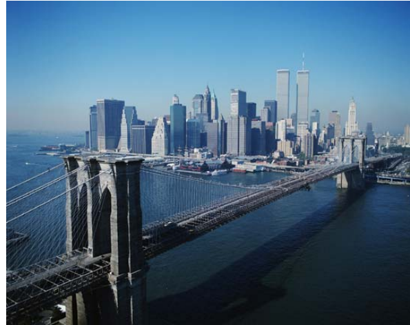
Figure XII.2.3.4.C This Bridge Supports Automobiles, Electric Trains and Pedestrian Traffic.
