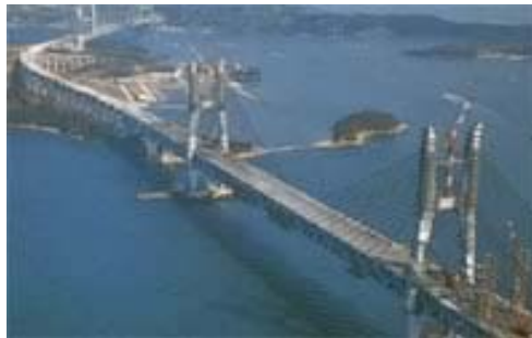
Figure XII.2.3.4.A The Seto-Ohashi Bridge supports 8 km of SEI's specially built cable.
