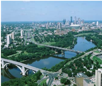
Figure XII.2.3.4.B These Bridges Support only Automobiles
