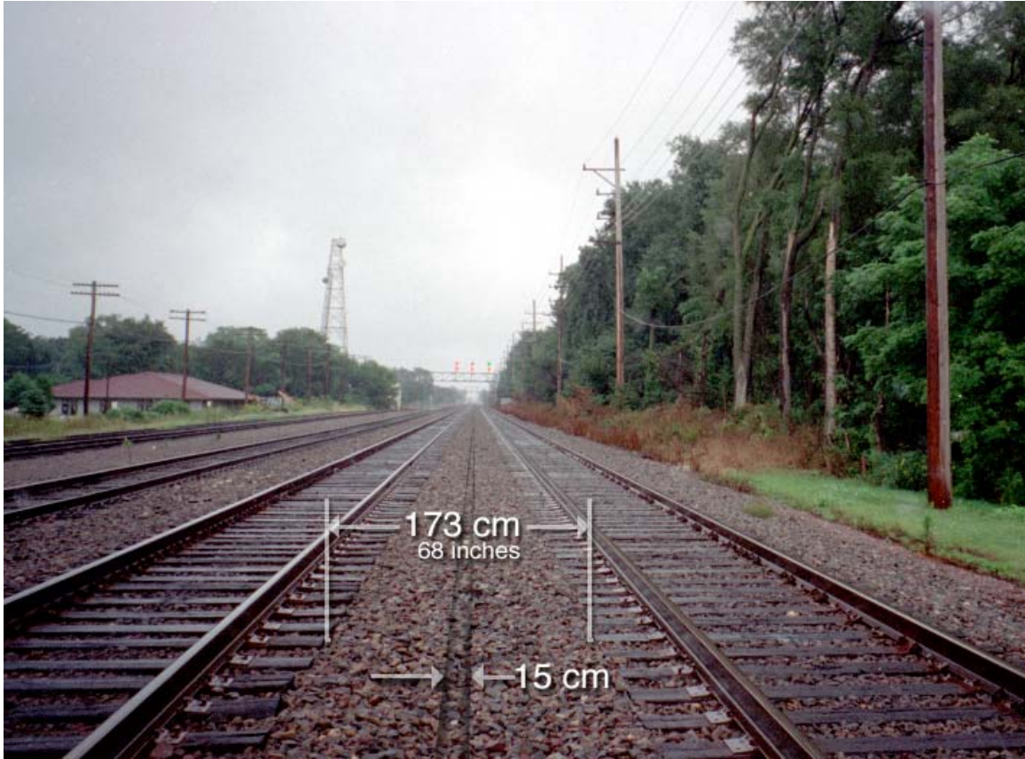
Figure XII.2.3.1 Looking From Suburbs, Along the Burlington Northern's Tracks, Toward the Center of Chicago
