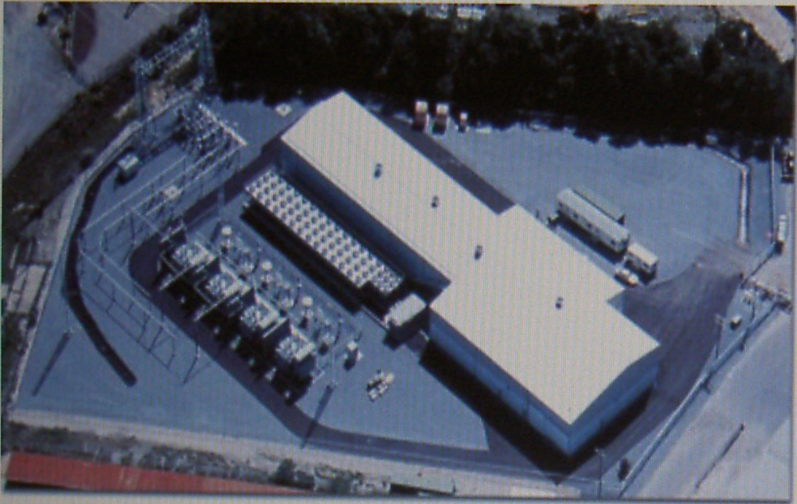
Shoreham converter station (Cross Sound Cable) 80m x 25m x 11m (Length x Width x Height)
