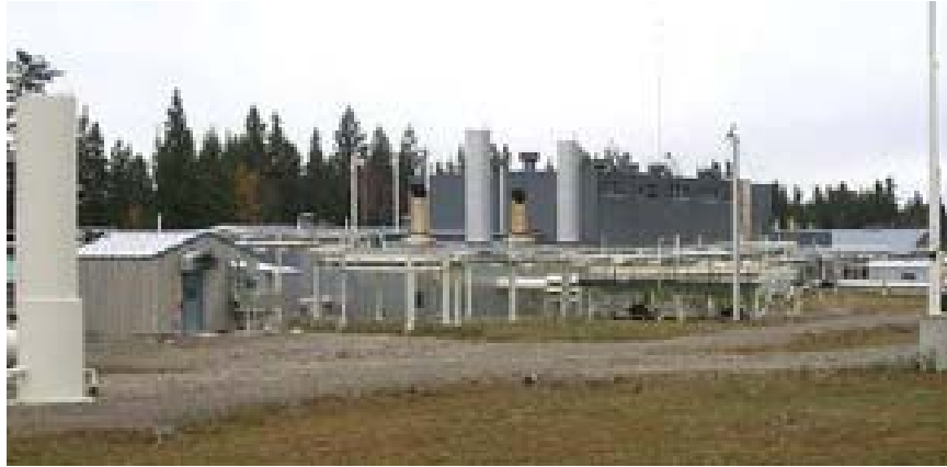
Figure 8-20 Pumping station for a natural gas pipeline
