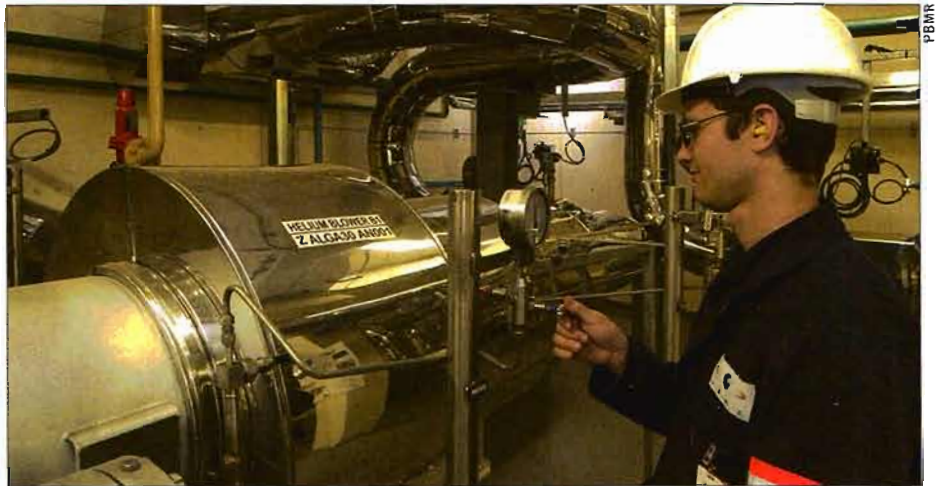
Pressure point The failed pebble-bed reactor in South Africa used helium as a coolant.
