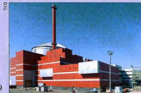
Leading the way The Olkiluoto 3 European pressurized water reactor currently being built on Olkiluoto Island in south-west Finland was, in 2005, the first to start construction.
