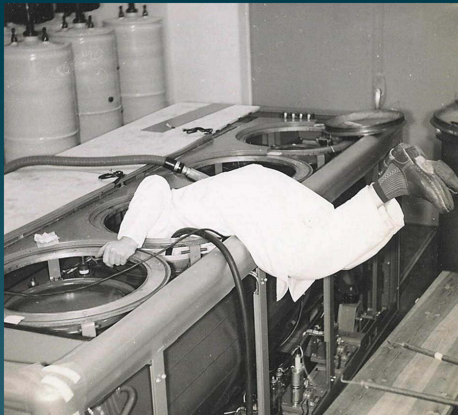
Anode Porcelains & Mercury Cathode Tank
