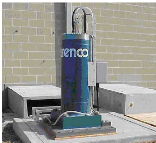
Figure 13-5 High-Speed Vertical-Shaft Composite Power Flywheel
