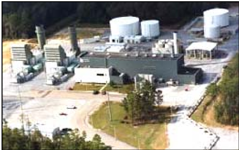
Figure 2 Underground CAES Plant, Alabama
