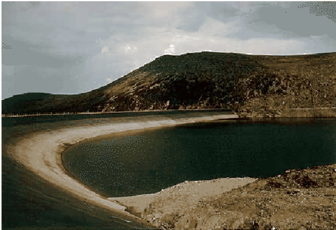
Figure 5.2: Upper reservoir of the Dinorwig plant in Wales.
