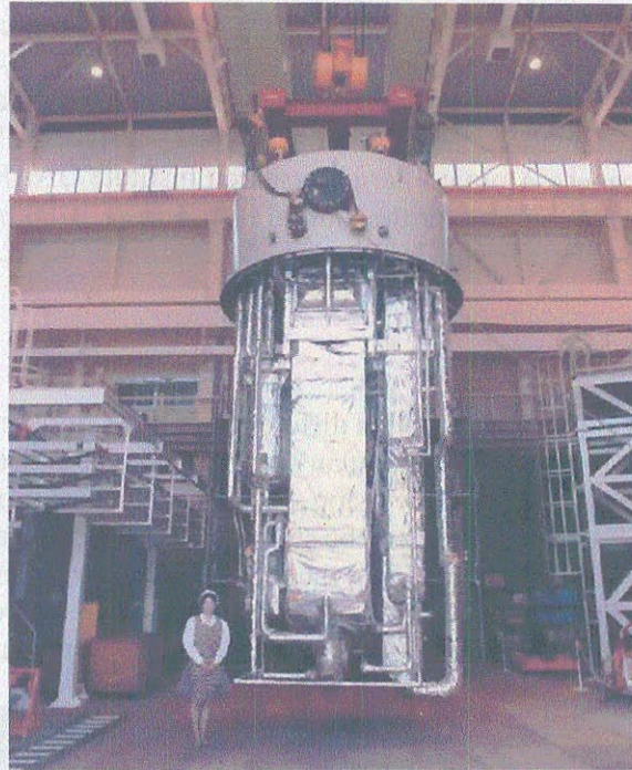
Figure 12-8 Large Liquid Helium Refrigerator (JAERI)
