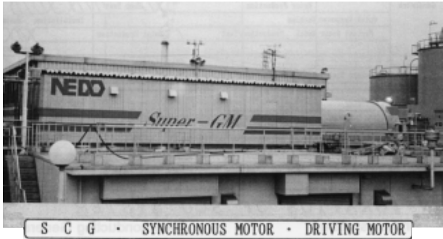
Fig. 2.1. External view of the Super-GM test facility at Osaka Power Station.
