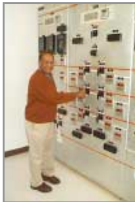
Electrical Control and Protection Panel for HTS Cables
