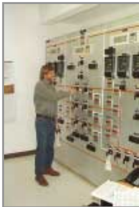
Electrical Control and Protection Panel for HTS Cables
