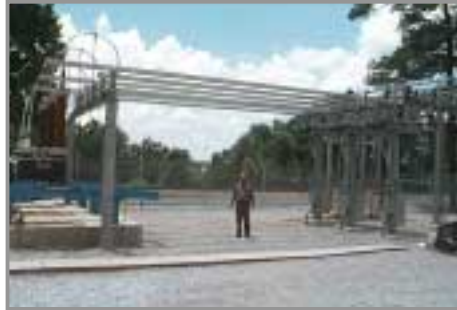
Future location of splice at 30-m test site.
