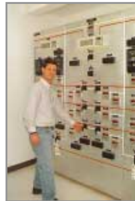
Electrical Control and Protection Panel for HTS Cables
